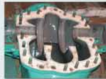
Reclaiming totally eroded surface
