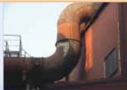
Coke Plant Pipe Elbow
